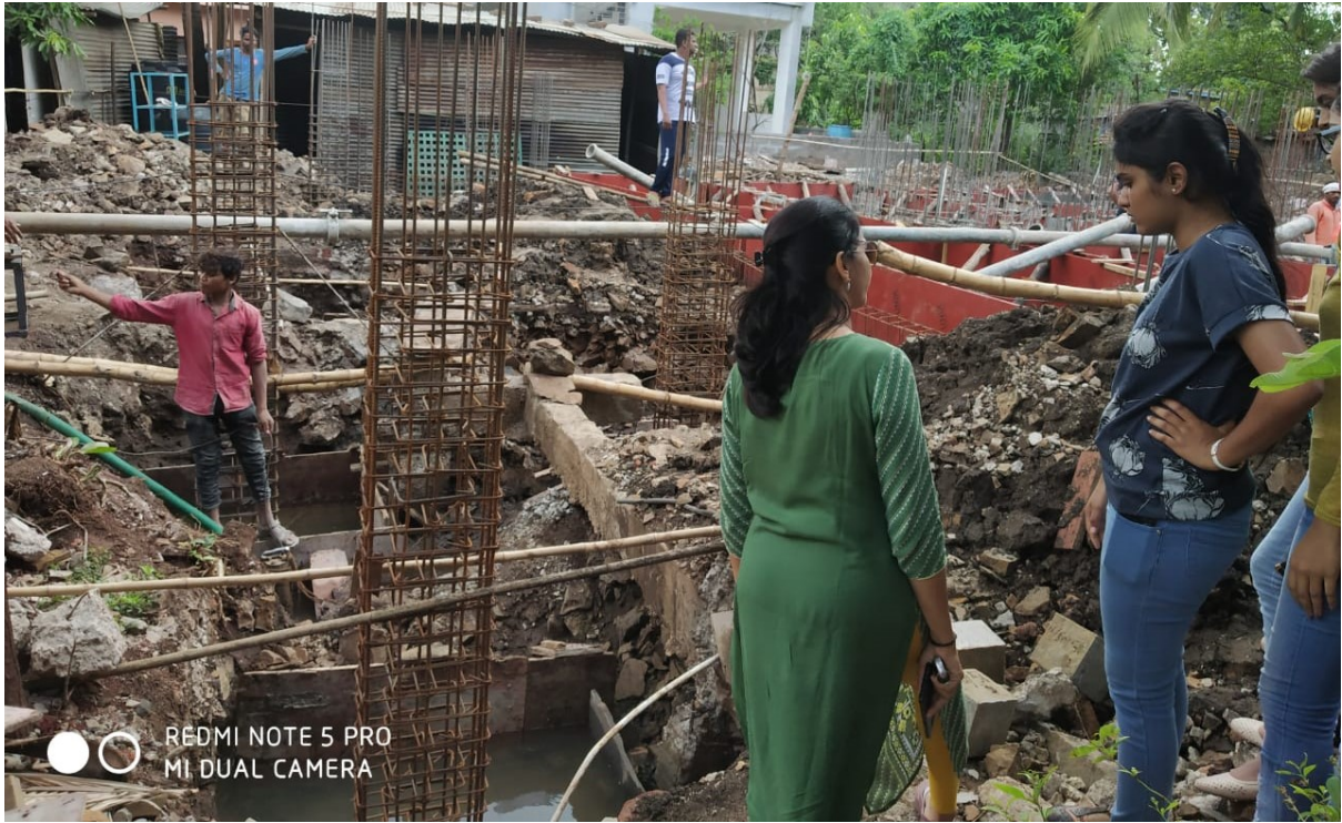
3 Students studying construction of foundations on site
