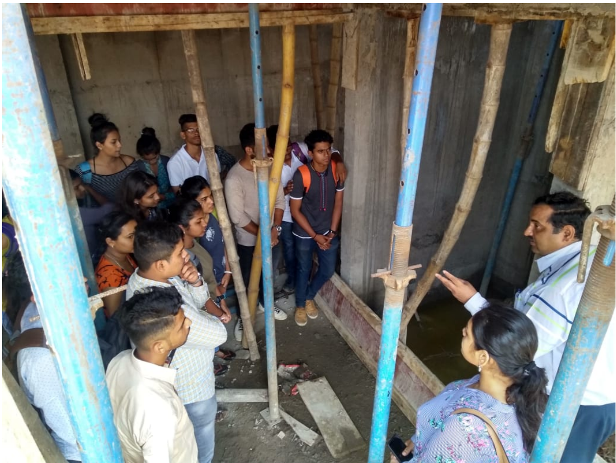
4. Students studying construction of Lift Pit on site.
