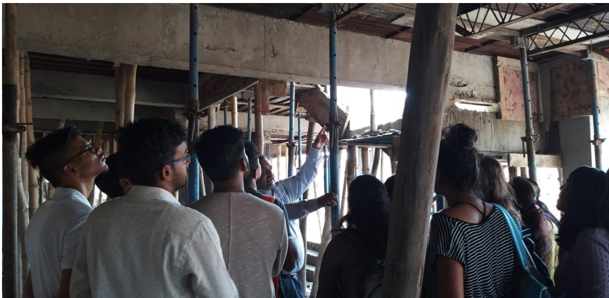
1. Retaining Wall and Basement Construction
