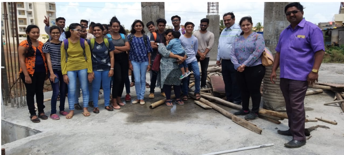
2. Students studying Column Construction and Reinforcement details on site
